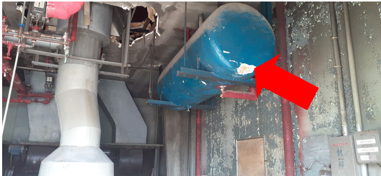
View of the above ground heater located in the storage shop #1 area in Building 1. (Samples 25 and 26). The piping insulation was found to contain 30% Chrysotile Asbestos (indicated by the red arrow).
