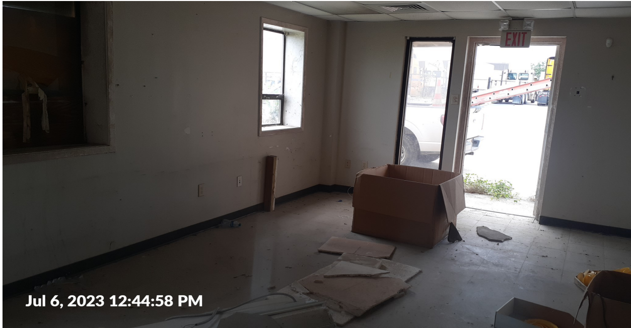
View of the utility room located in the northwest part of Building 6 (Samples 01 & 02).
