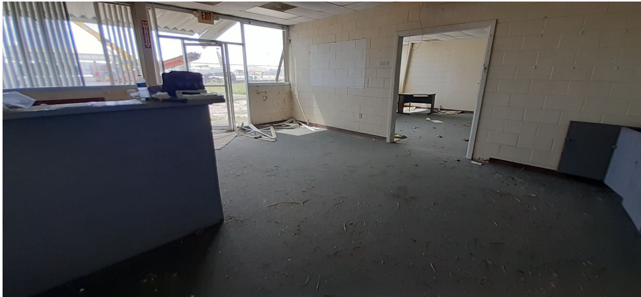
View of the Reception Lobby and Offices in Building 1 (Samples 01 & 02).
