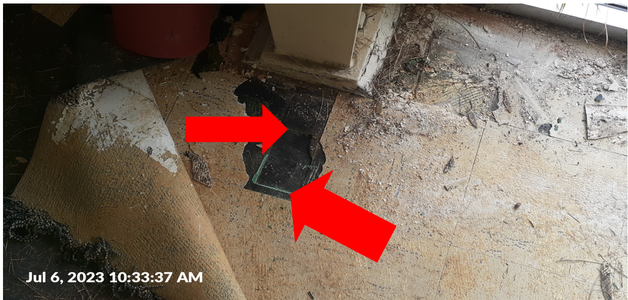
View of the black mastic and green 12" x 12" vinyl floor tile in Building 1. The black mastic was found to be positive for asbestos (3% Chrysotile Asbestos) (Samples 01 & 02). The green vinyl floor tile was found to be 7% Chrysotile Asbestos (Samples 03 & 04).
