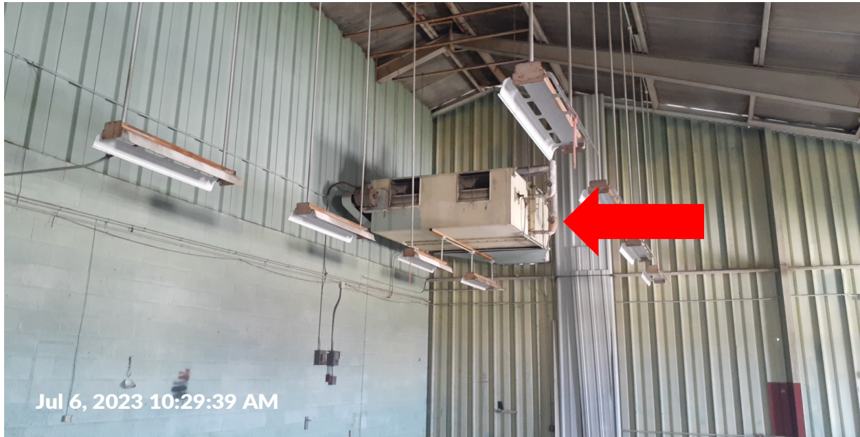
View of the above ground heater located in the storage shop #1 area in Building 1. (Samples 25 and 26). The piping insulation was found to contain 30% Chrysotile Asbestos (indicated by the red arrow).
