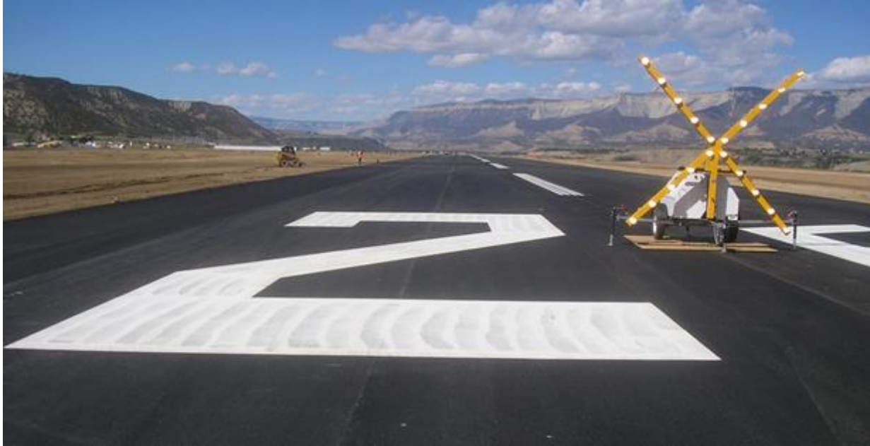
Figure 2-7. Lighted X at Night
